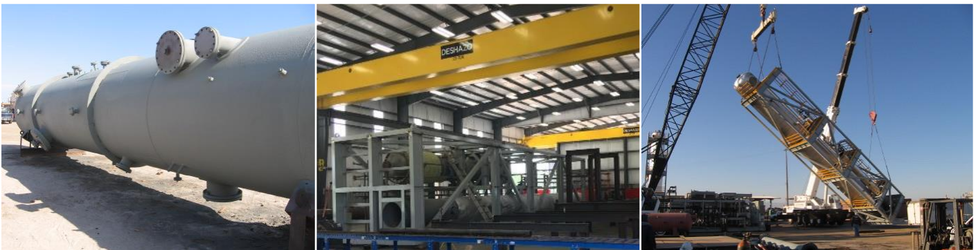
Figure 4: Horizontal Construction of Pressure Vessels and Columns
